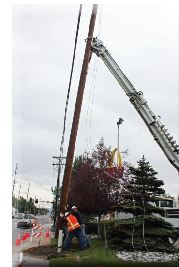
Chugach crews replaced a wood structure broken in a car accident.
