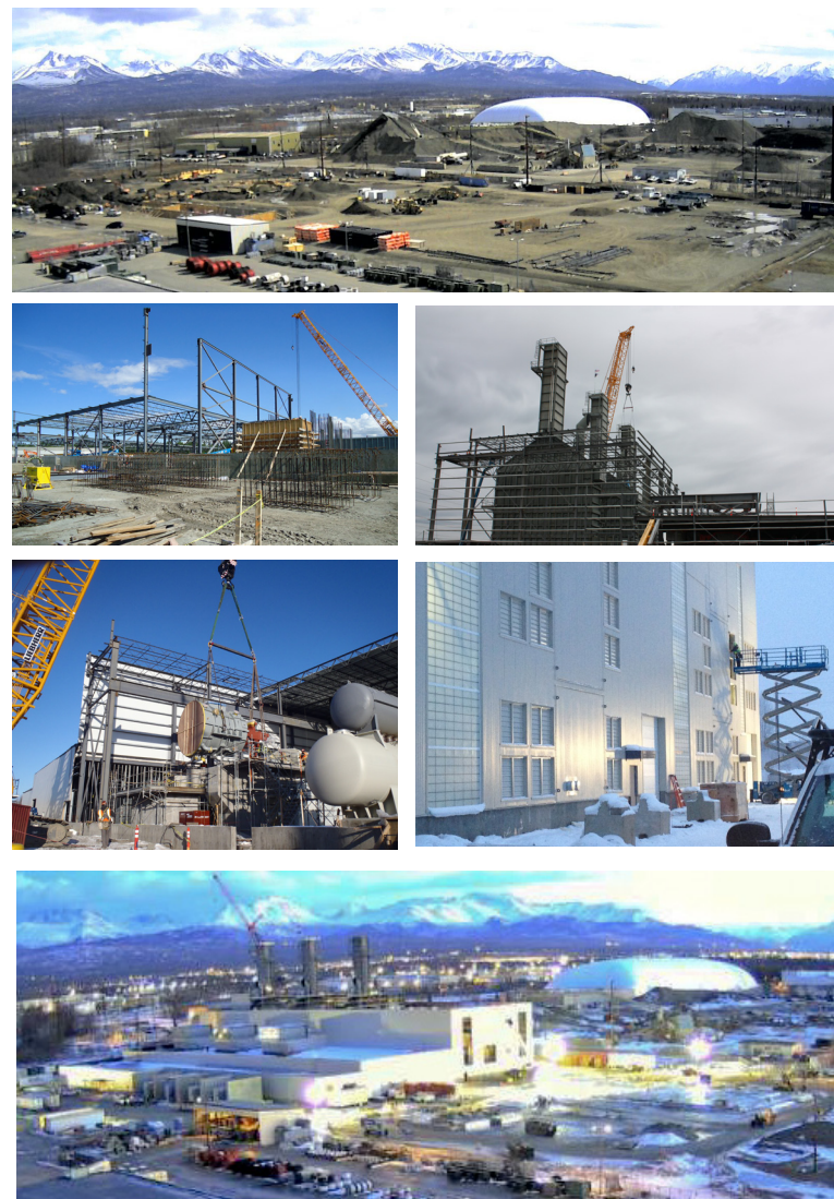
Above: Southcentral Power Project construction
