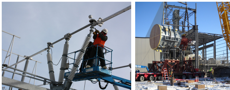
Top left: Beluga Unit 5 turbine rotor disassembly Top right: Beluga Unit 5 inspection Bottom left: Pt. McKenzie maintenance Bottom right: Setting the steam turbine generator at SPP
