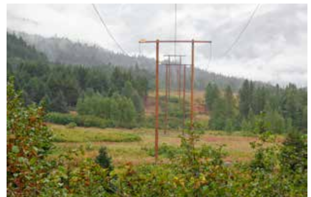
Chugach continued supporting unification of the Railbelt transmission grid, working with other utilities toward the goals of creating both a regional transmission company (Transco) and a Unified System Operator.
