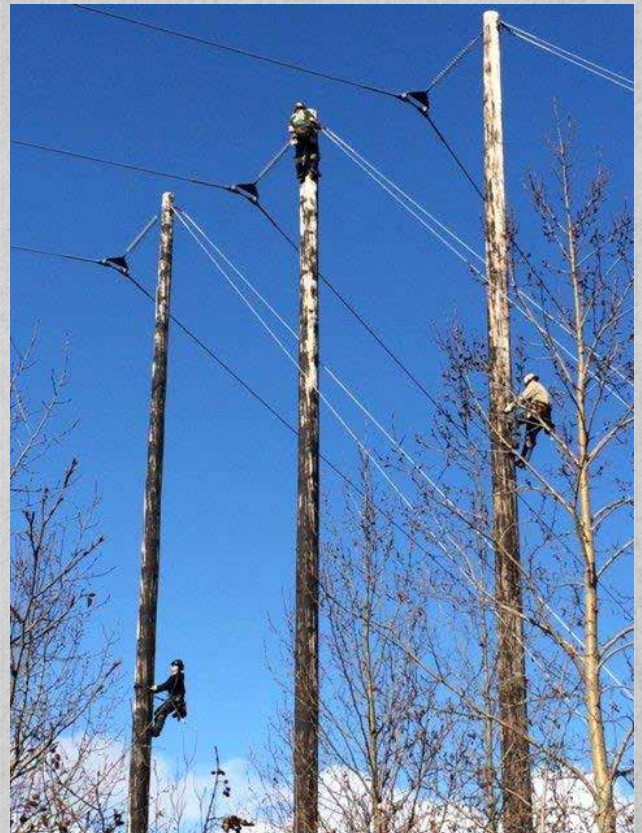
Crews conducting a climbing inspection of a 3-pole angle structure on the 115-kilovolt transmission line between Girdwood and Portage.
