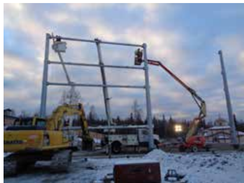
Construction of the Hane Substation continued throughout the winter.
