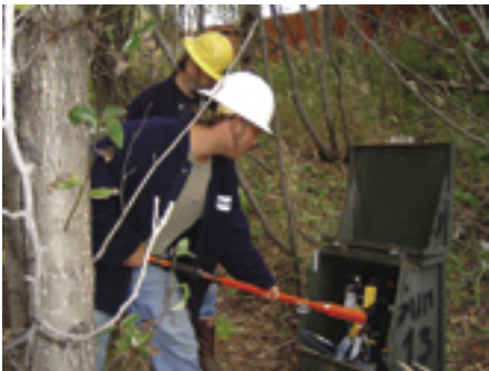
The Power Delivery group also maintains underground distribution lines and uses a cable injection technique for extending the life of aging underground systems. In 2003, Power Delivery crews injected 31,400 feet of underground distribution cable in six subdivisions, including Bayshore West, Oceanview North, and Stonegate Townhouse, extending the life of the underground cable by 15-20 years.
