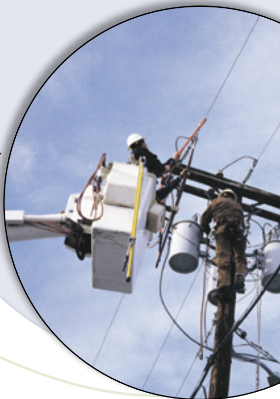
Chugach linemen installing a bank of transformers on an overhead line.
