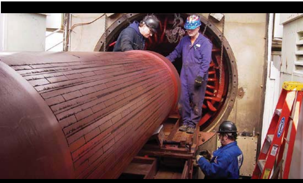
Chugach completed a generator inspection on Beluga Unit No. 5 in May.
