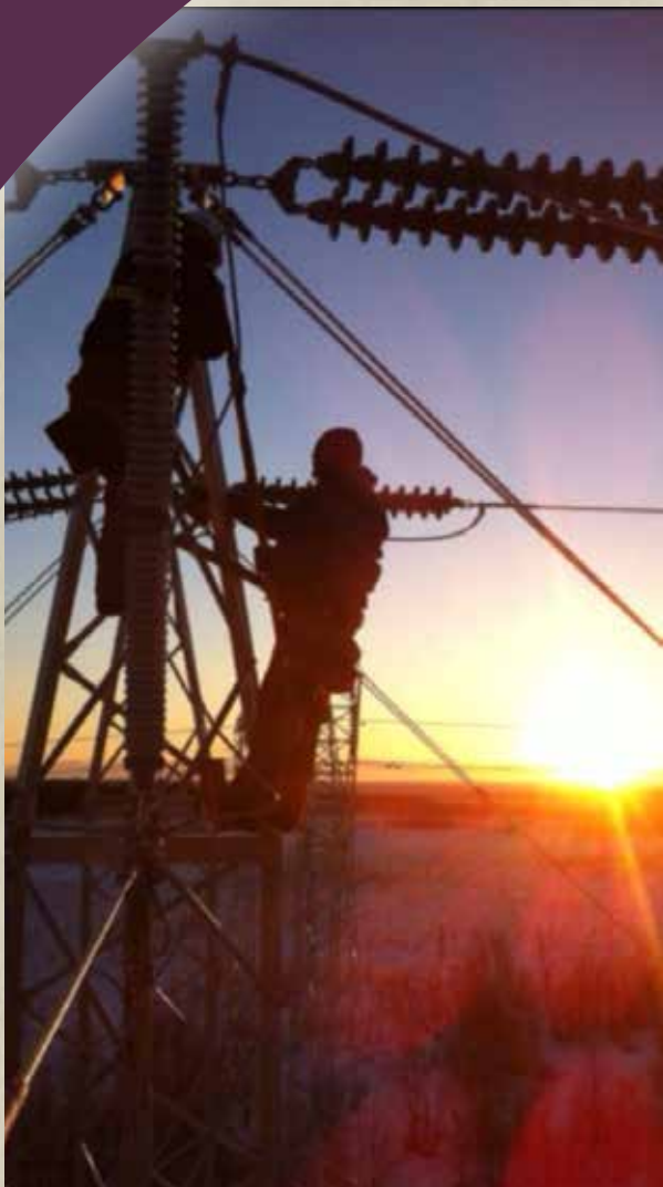
Lineman periodically do climbing inspections of Chugach's transmission structures.
