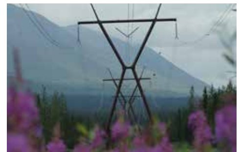
Chugach executed a gas purchase contract and a power sales agreement for economy energy to Golden Valley Electric Association for a two-year period beginning April 1, 2013.
