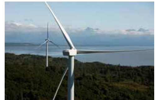
Chugach took its first full year of energy from the Fire Island Wind Project in 2013, using its hydro resources to manage wind variability. The project had a 29 percent capacity factor, producing 49,525 megawatt-hours of energy.
