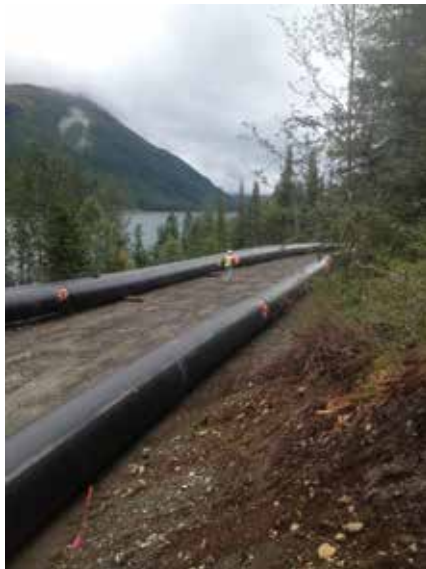
A diversion structure (left) and more than 2 miles of 48-inch pipeline (center) will divert water from Stetson Creek into the Cooper Lake reservoir, where a siphon (right) will convey water into the Cooper Creek drainage below the dam.
