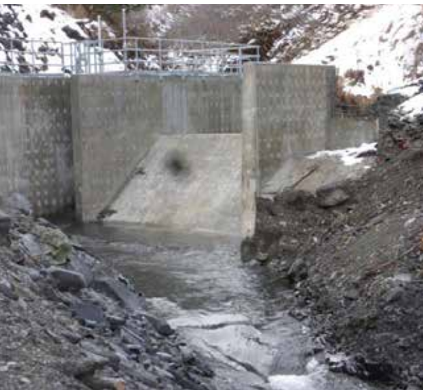
A diversion structure (left) and more than 2 miles of 48-inch pipeline (center) will divert water from Stetson Creek into the Cooper Lake reservoir, where a siphon (right) will convey water into the Cooper Creek drainage below the dam.
