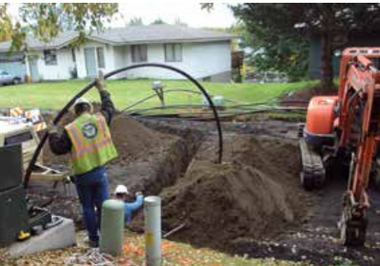
Counter-clockwise from top: A project to install a pair of underground 34.5-kilovolt feeder circuits from the Retherford Substation was completed in 2014. Chugach continued to replace existing overhead circuits and failing cable with new underground lines in 2014. Corrosion was addressed at the foundation of a transmission tower along Turnagain Arm. Crews installed a new overhead crossing at the Chuitna River, driven by damage from 2012 flooding. A contractor cleared the alignment for the future rebuild of a section of 115-kv transmission line near the community of Indian.
